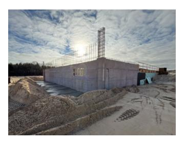
In terms of implementation, approximately **600 cubic yards of Bio-San concrete** were used in the headworks of the new Wastewater Treatment Facility (WWTF), specifically in the **screening channels, grit chamber and hauled waste tanks**. This application improves both the durability and efficiency of the filtration system. An additional **500 cubic yards will be used in the main lift station**, which transfers wastewater from the existing facility to the new plant.
