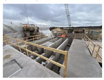
To enhance the durability and performance of the construction, Xypex's Bio San was selected to combat Microbial Induced Corrosion (MIC). MIC refers to the deterioration of materials, particularly metals and concrete, caused by the activity of microorganisms. These microorganisms thrive in  $H_2S$  environments, generating acids and sulphates which corrode concrete.
